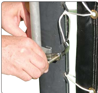
Step 4: Push the screw toward the net post and turn the screw to tighten the clamp band.
