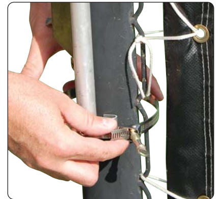
Step 3: Secure the Mount clamp by inserting the band into the screw assembly.
